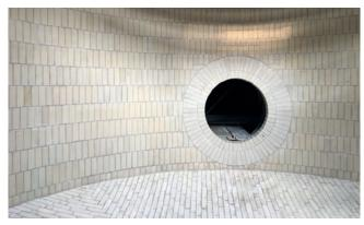
Brick lined pump tank in a sulphuric acid plant – Asplit HB Mortar
